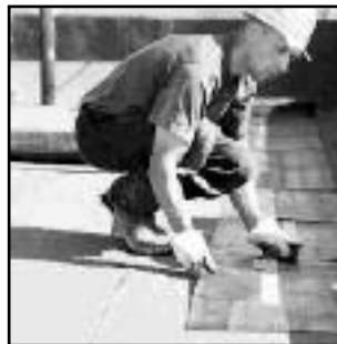
FLAT TOP ROOF
