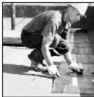
FLAT TOP ROOF
