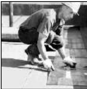
FLAT TOP ROOF
