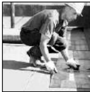
FLAT TOP ROOF
