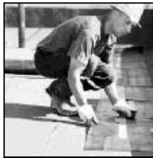
FLAT TOP ROOF
