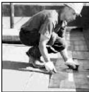
FLAT TOP ROOF
