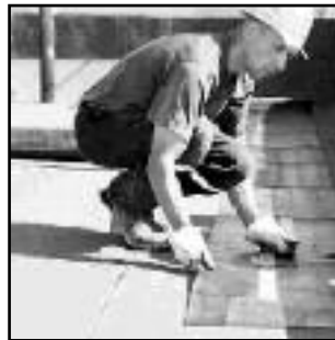
FLAT TOP ROOF
