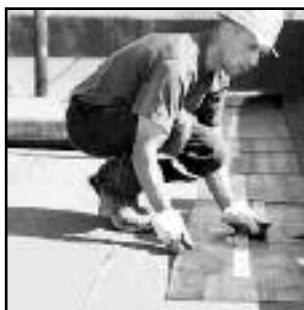
FLAT TOP ROOF
