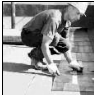
FLAT TOP ROOF
