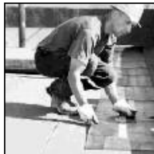
FLAT TOP ROOF
