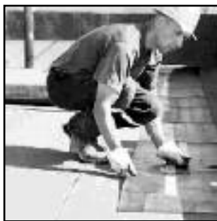
FLAT TOP ROOF
