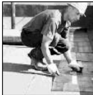
FLAT TOP ROOF
