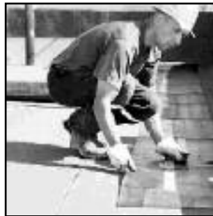
FLAT TOP ROOF
