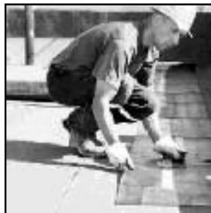
FLAT TOP ROOF
