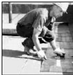
FLAT TOP ROOF
