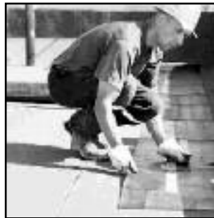
FLAT TOP ROOF
