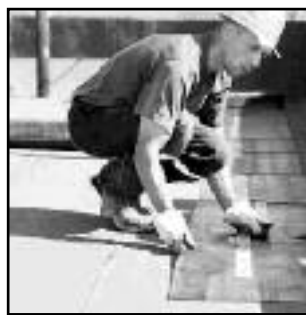
FLAT TOP ROOF
