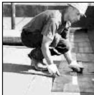
FLAT TOP ROOF
