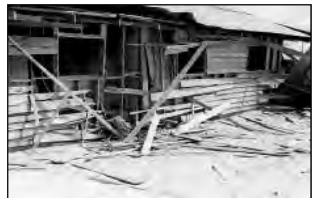
The badly damaged Non-Commissioned Officer (NCO) barracks hooch that Gilbert Secor shared with Ray Steele and Cleveland Graham at Marble Mountain on August 23, 1968.
