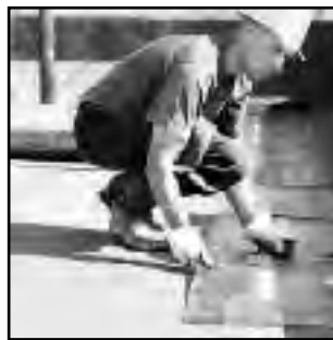
FLAT TOP ROOF
