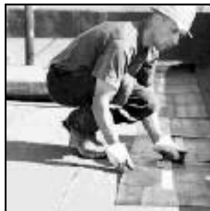
FLAT TOP ROOF
