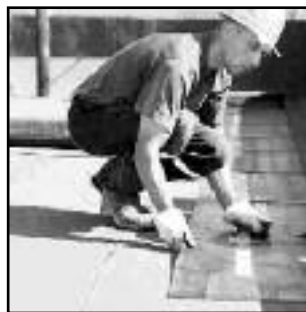
FLAT TOP ROOF
