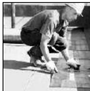
FLAT TOP ROOF
