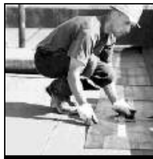
FLAT TOP ROOF
