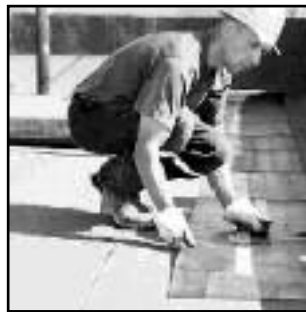
FLAT TOP ROOF
