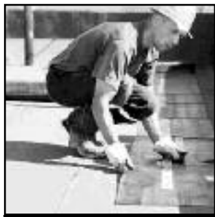
FLAT TOP ROOF
