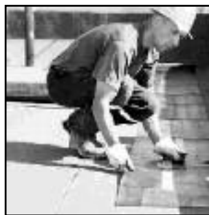
FLAT TOP ROOF
