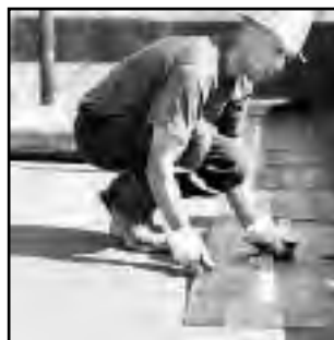
FLAT TOP ROOF
