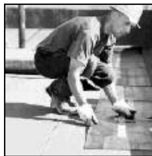
FLAT TOP ROOF
