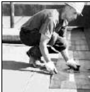
FLAT TOP ROOF
