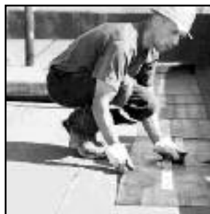
FLAT TOP ROOF
