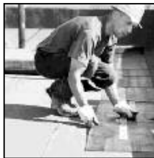
FLAT TOP ROOF
