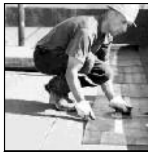
FLAT TOP ROOF
