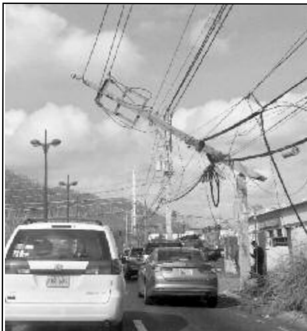
(above) Heavy traffic, downed utility pole.
