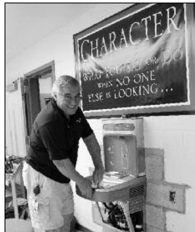
(above) Skilled maintenance worker Ralph Circelli installs environmentally-friendly water
